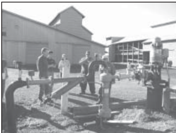
New irrigation system at Annen Farms
