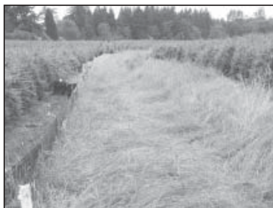
Sediment fencing and installed grass filter strip.
