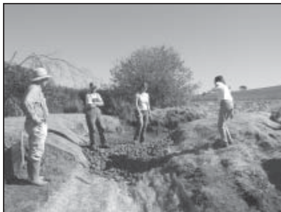
Inspecting the new sediment basin.
